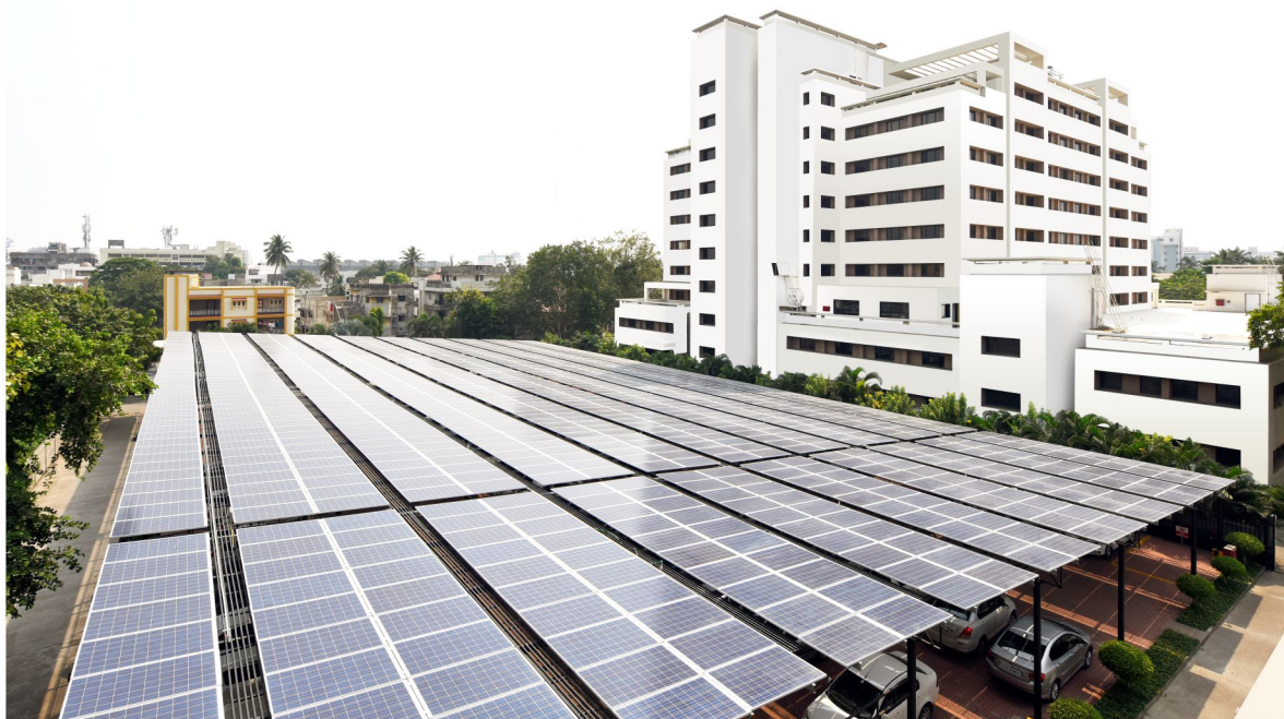
20% of the factory's power requirement is fulfilled by the solar panels installed at Venus Jewel.
